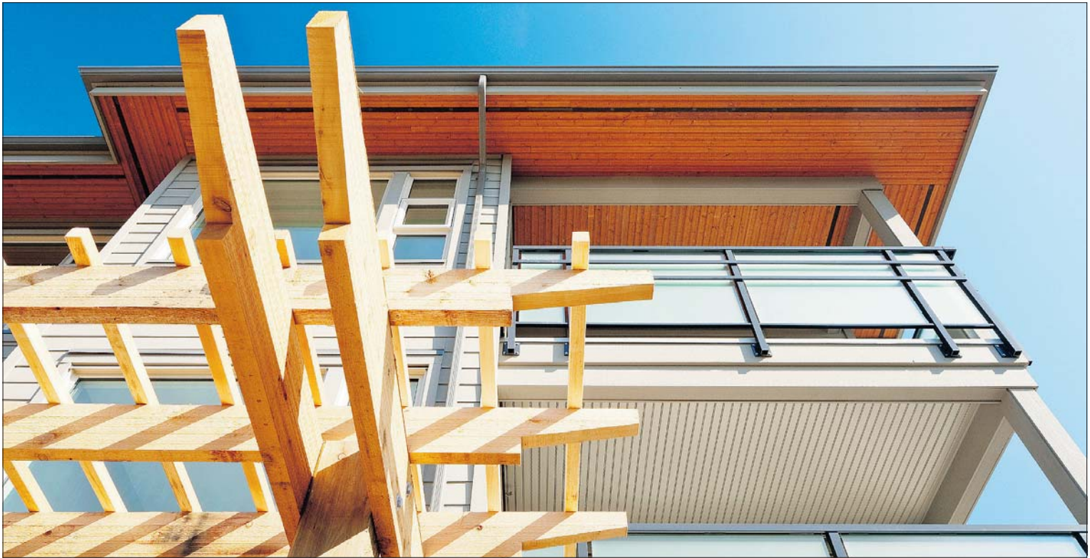
District Crossing new-home project in North Vancouver, a product of architect Raymond Letkeman marked by posts and beams topped by crossed purlins. — SUBMITTED PHOTOS
